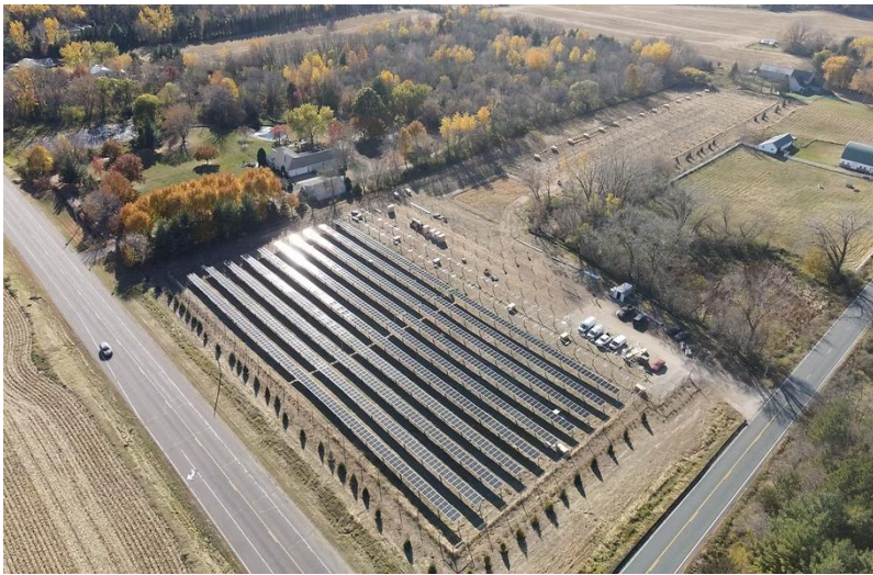
Lake Elmo Solar Garden, outside of St. Paul, Minnesota. Photos from Cooperative Energy Futures
